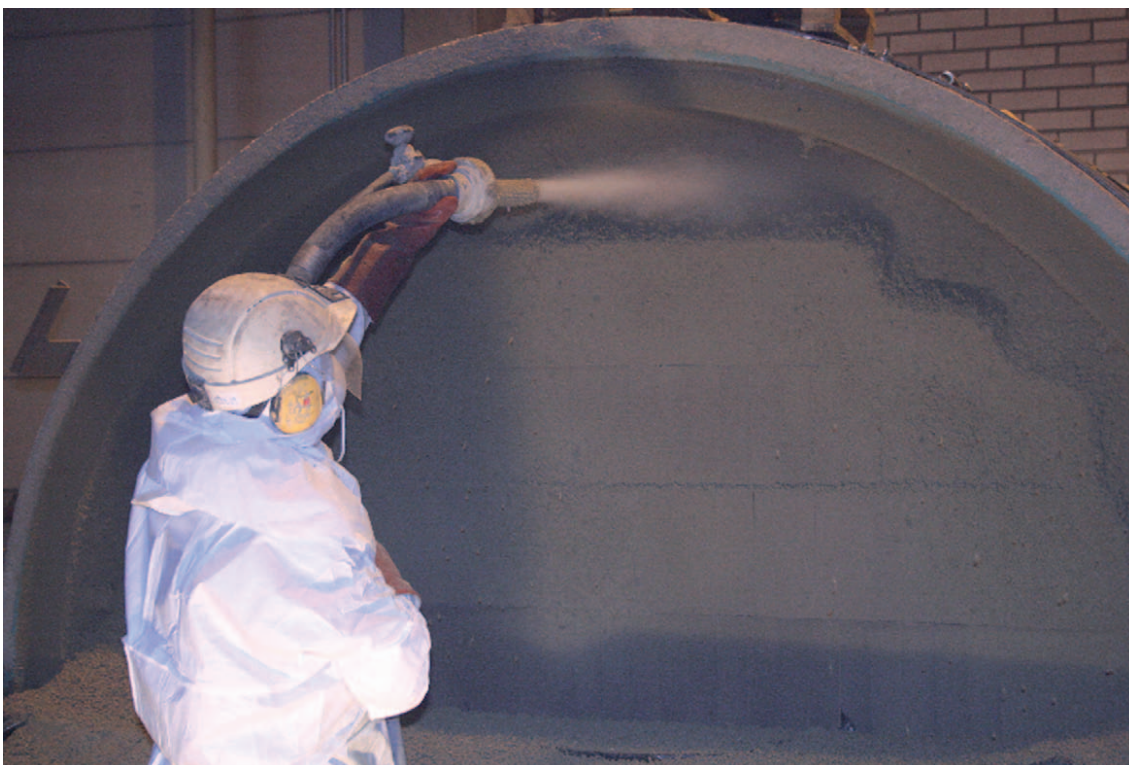
Testing of the tunnel backfill operation.
